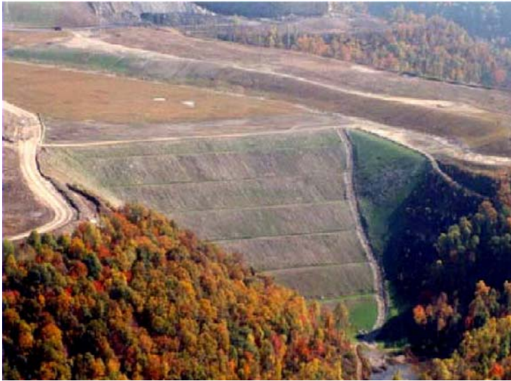
Figure 1. A typical valley fill. Note across-face terraces and rock drain along the side. Many fills also have a center drain. The original stream bed emerges at the toe of the fill in the lower right.
